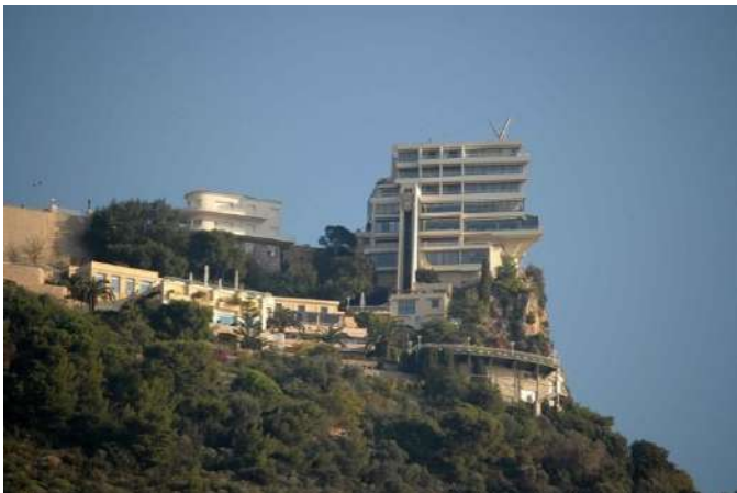
2017: just before the demolition of the Vista Palace Hotel, formerly Vistaéoro.
